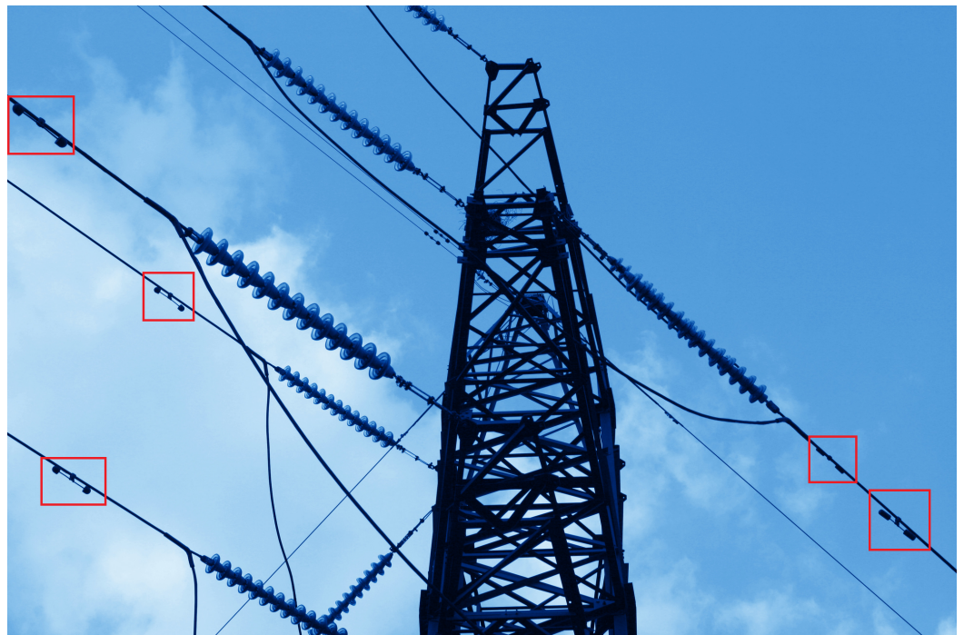
Figure 16. Shock absorbers on power lines.
